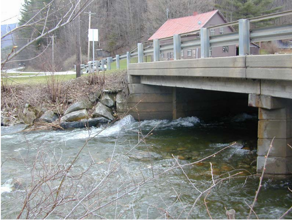
East (downstream) side of bridge, looking south
