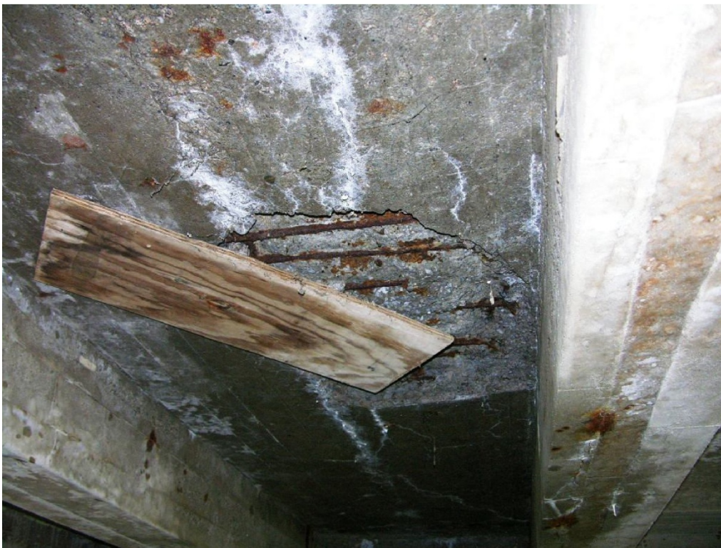
Deck deterioration
