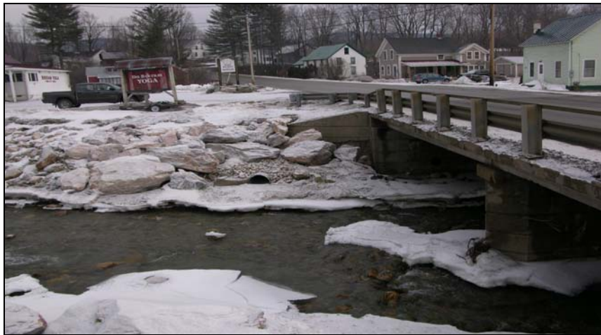
Figure 6: CMP Outlet at Northeast Wingwall
