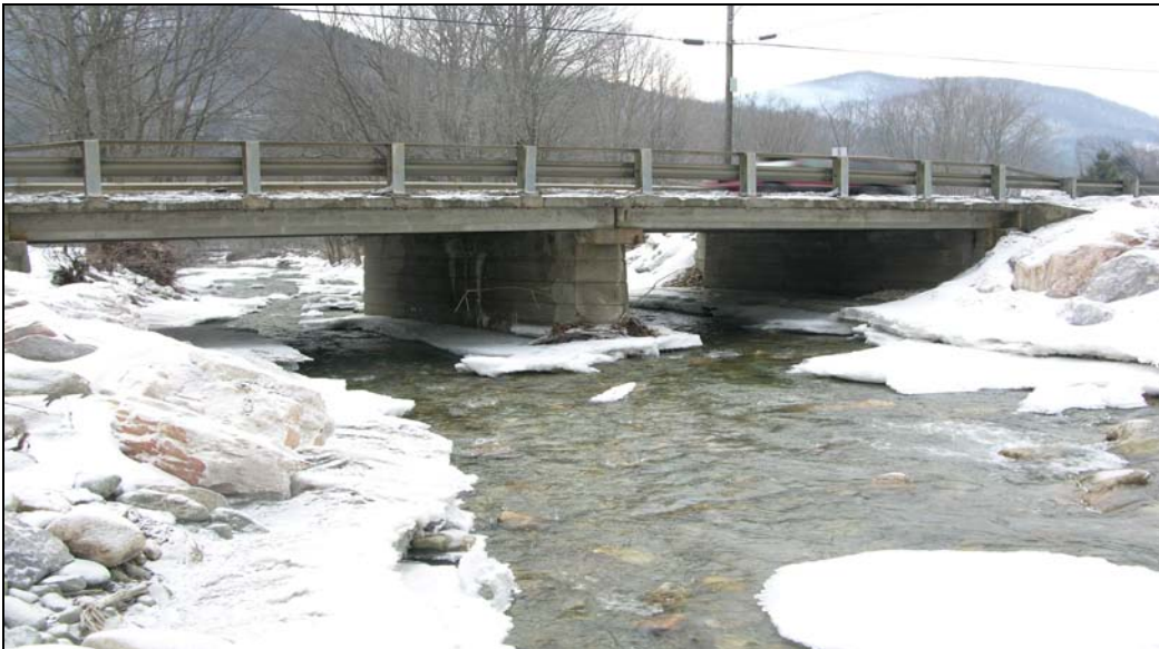
Figure 1: VT 100, Bridge 126 over the Second Branch of the Tweed River
