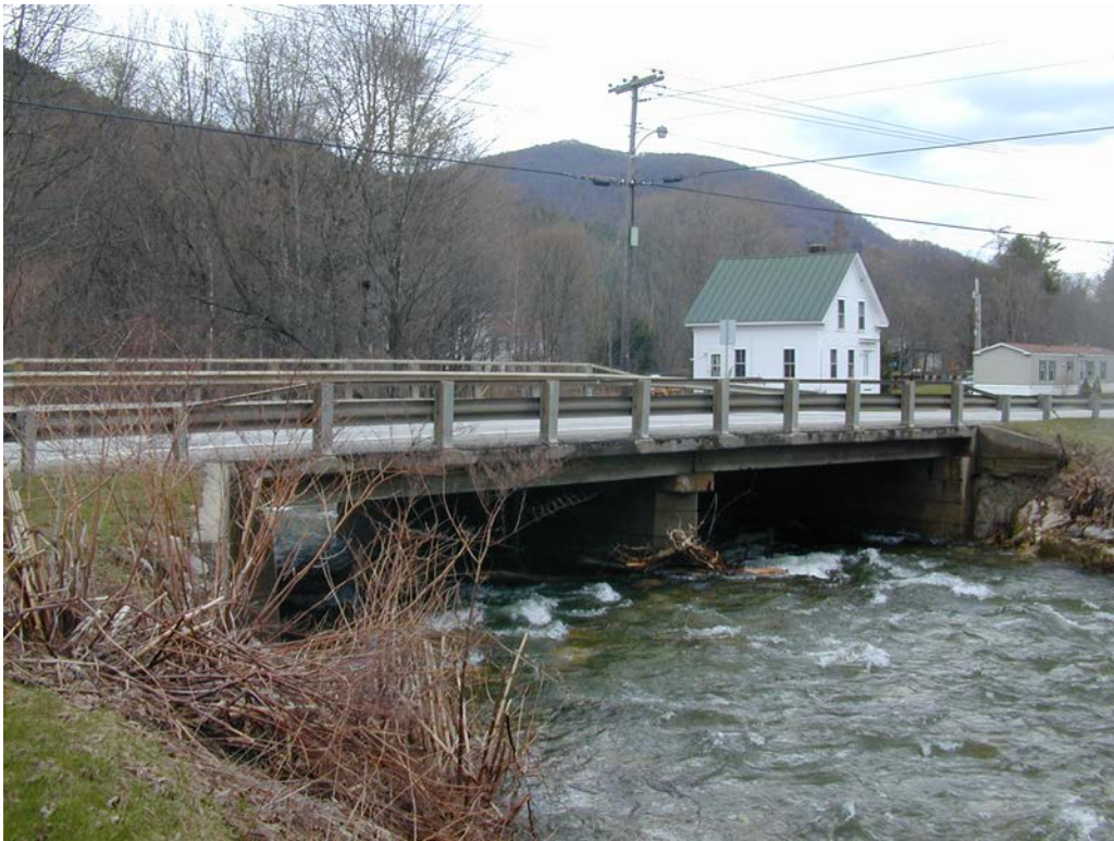
West (upstream) side of bridge looking south
