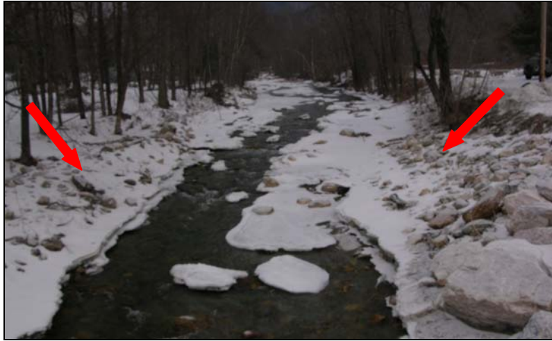
Figure 4: Possible Waterway Restriction due to Boulder Debris (Upstream)
