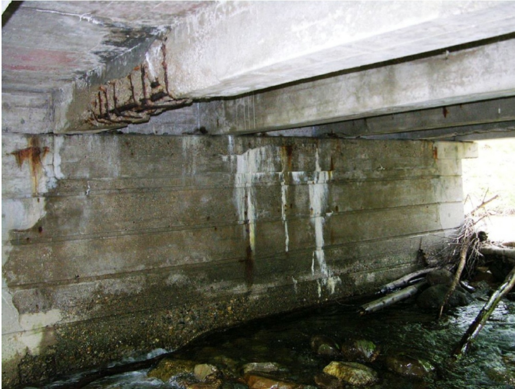
Abutment and tee-beam deterioration
