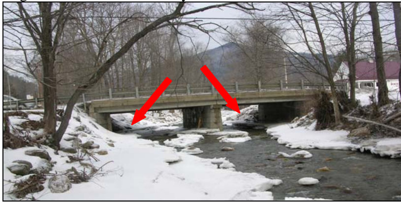
Figure 5: Possible Waterway Restriction due to Large Rip-Rap
