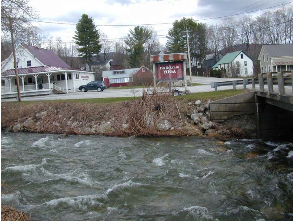
West (upstream)side of bridge looking north
